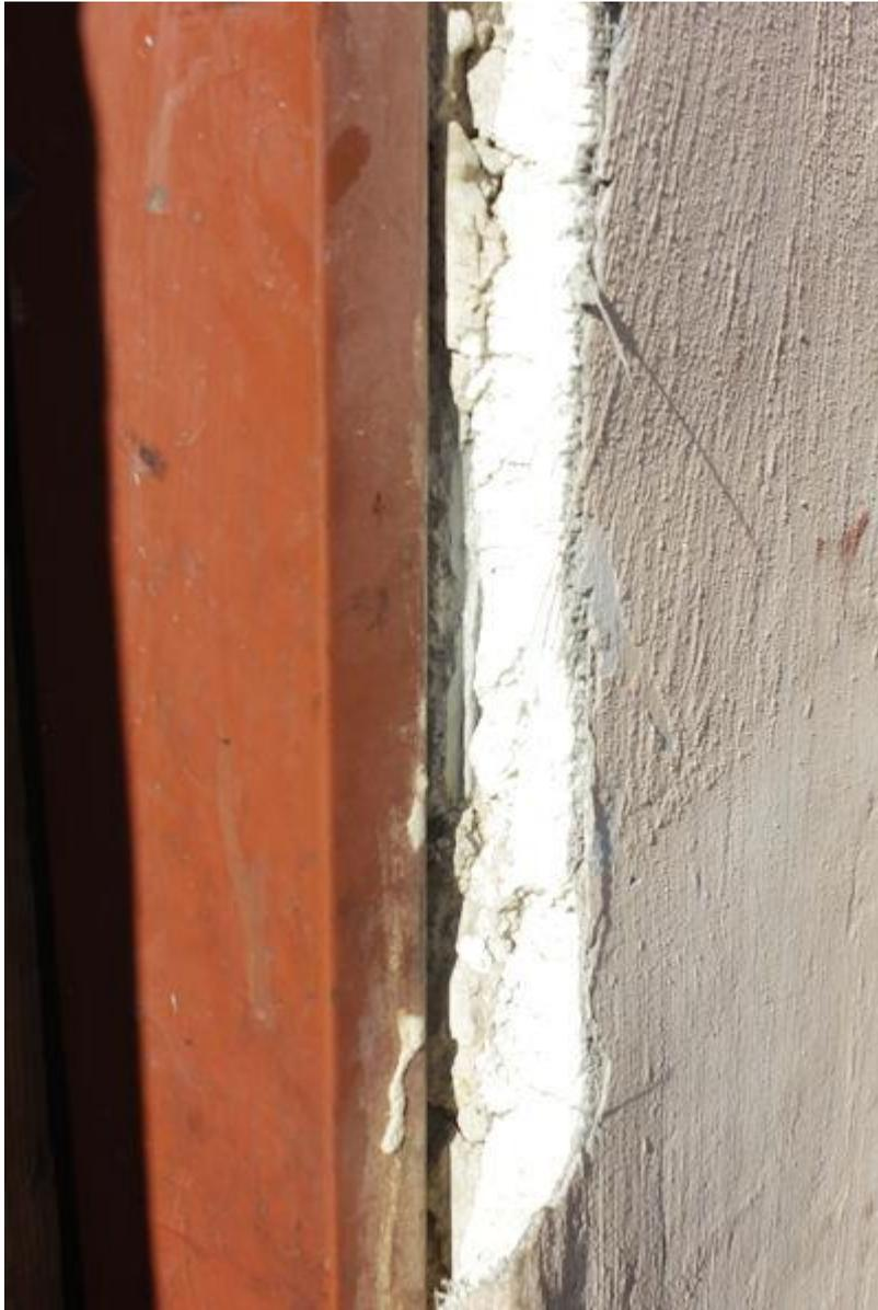
Styrofoam cladding coming away from brickwork
